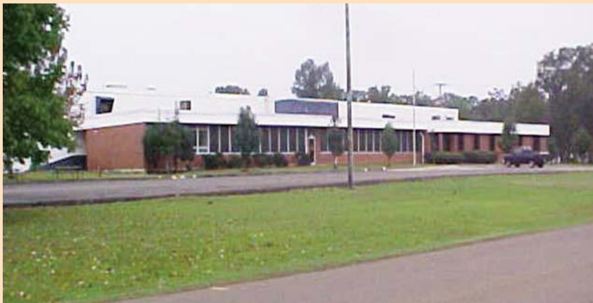
Amory MS facility
